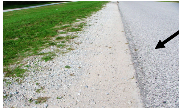
Example of bad drainage with road edge crumbling
